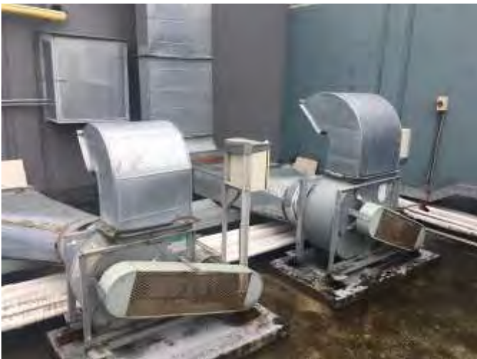
Exhaust Ventilation Blowers
