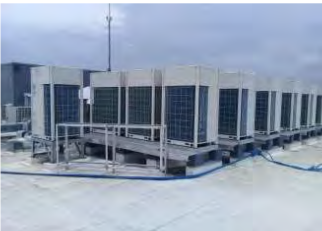
VRF Air Conditioning System at rooftop
