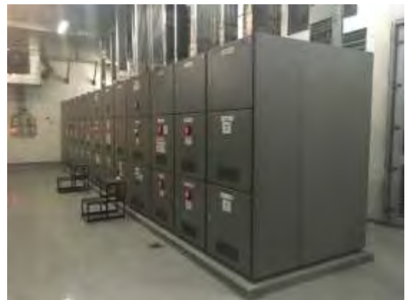
Low Voltage Switchgear
