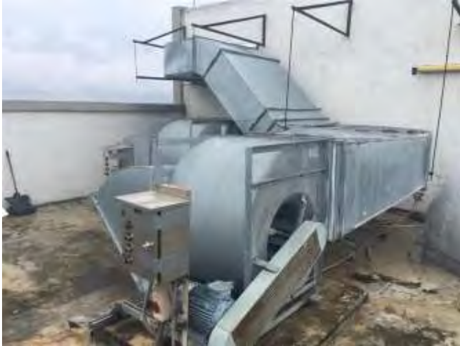
Pressurization Blower Fans
