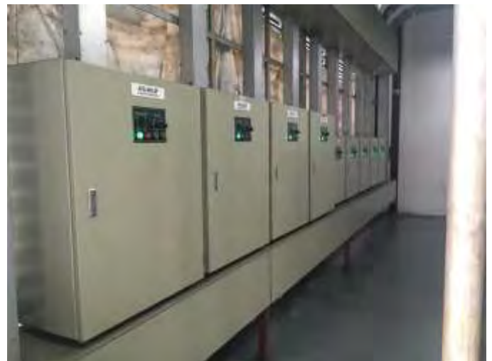
Automatic Transfer Switches
